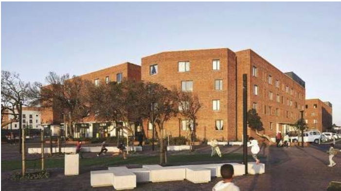
Conradie Park, Cape Town, South Africa. Photo: Sean Gibson / dhk Architects.
