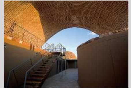
Interior View. Google Maps/visi.co.za
