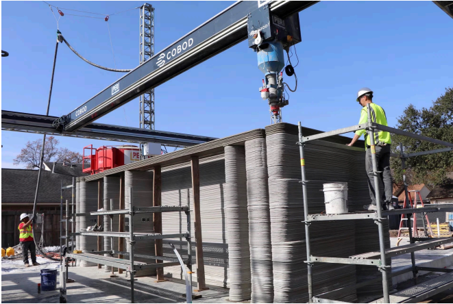
3D printing in construction. Image Credit: Google/parametric-architecture.com
